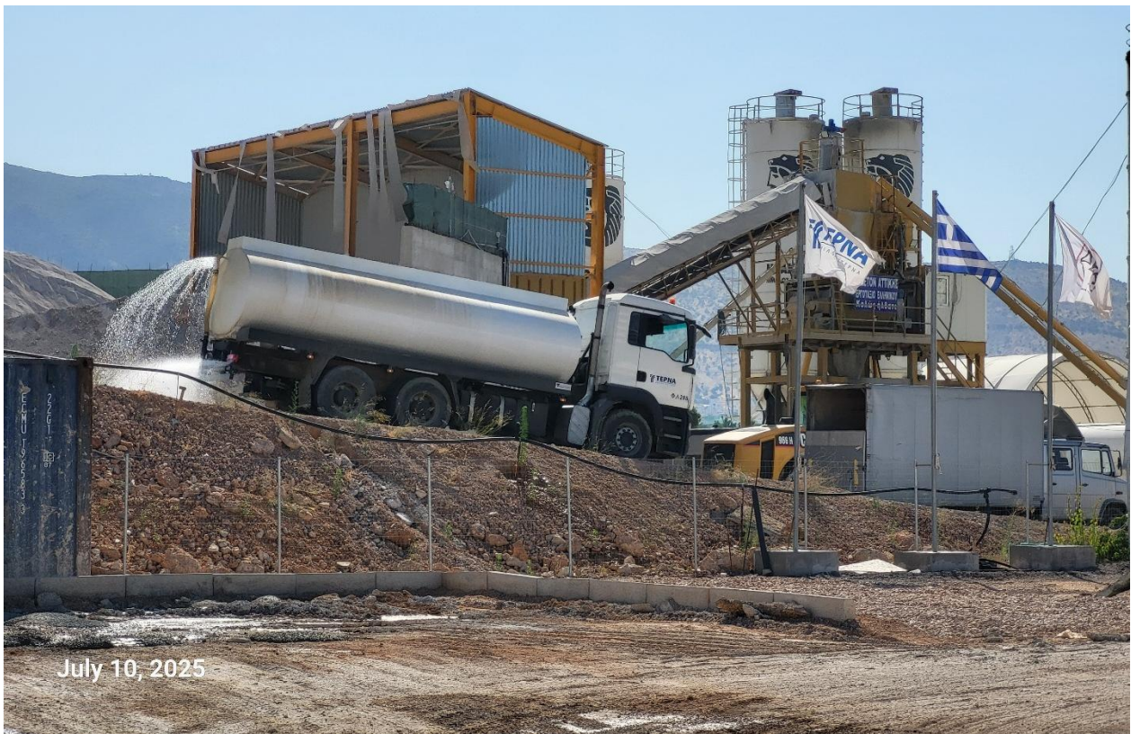
Figure 2.4-6: Wetting of concrete batching plant soil terrain as a mitigation measure for dust prevention
