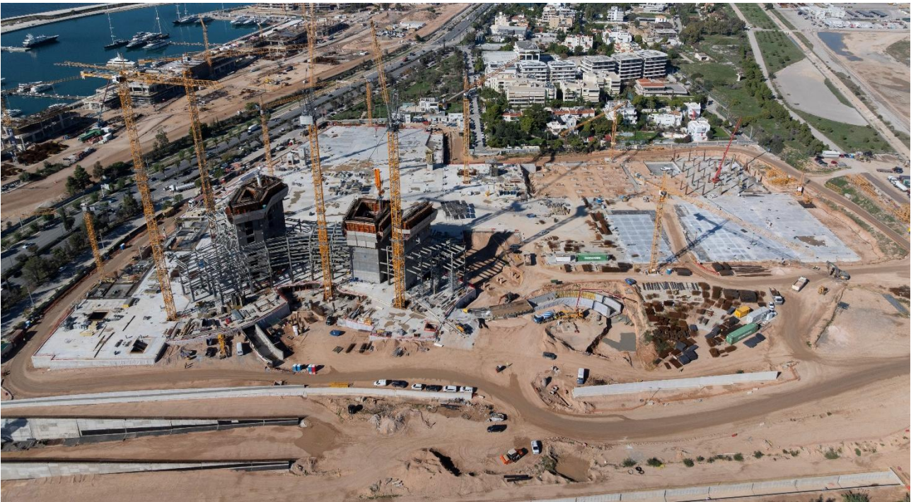
Figure 1.2-2: Construction site of the IRC Hellinikon
