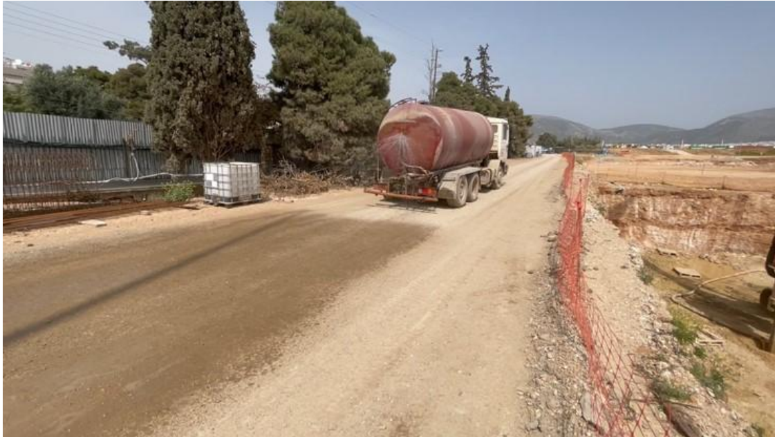
Figure 2.4-3: Wetting of unpaved roads as a mitigation measure for dust prevention
