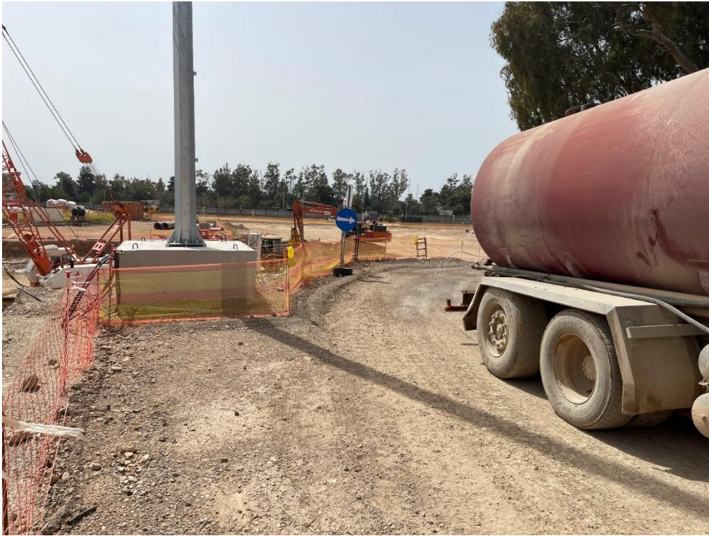
Figure 2.4-5: Wetting of unpaved roads as a mitigation measure for dust prevention
