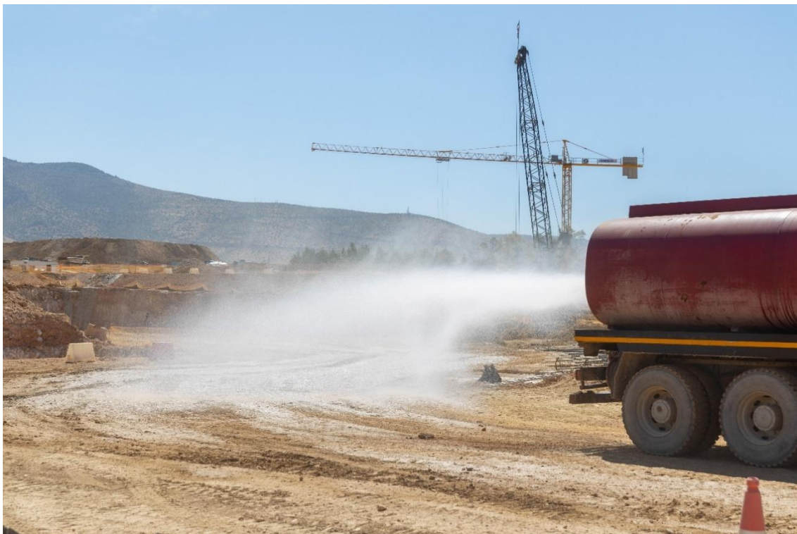
Figure 2.4-3: Wetting of unpaved roads as a mitigation measure for dust prevention
